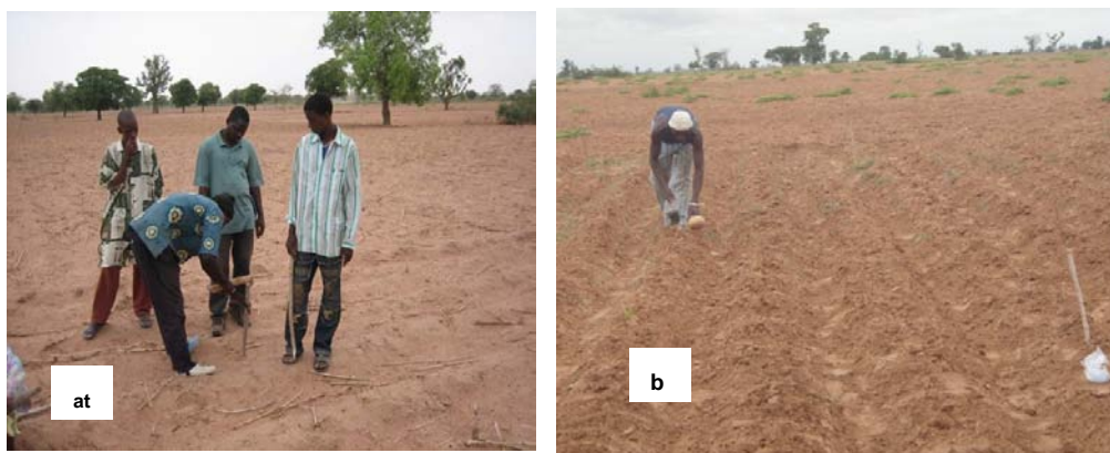
Photo 3: Staking contour using picket 40-50 cm long The survey of the contour line will start from the highest point of the field to be treated. The distance between the stakes will be up to 10 m, and it will be reduced if the shape of the contour is complicated (Figure 3).
